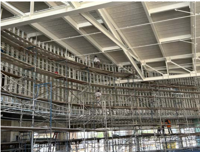
Natatorium Soffit Framing
