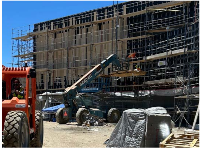
GFRG Install On South Elevation
