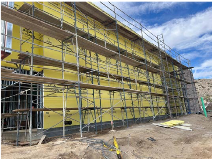
Segment 'A' Exterior Sheathing
