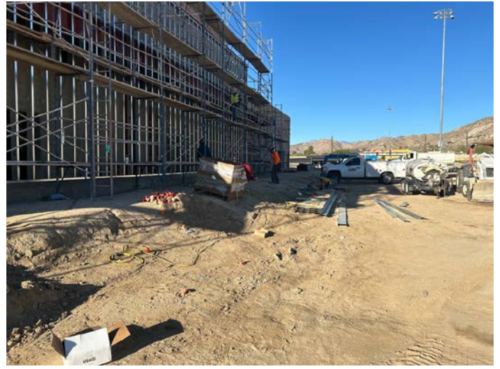
Segment 'A' Exterior Framing
