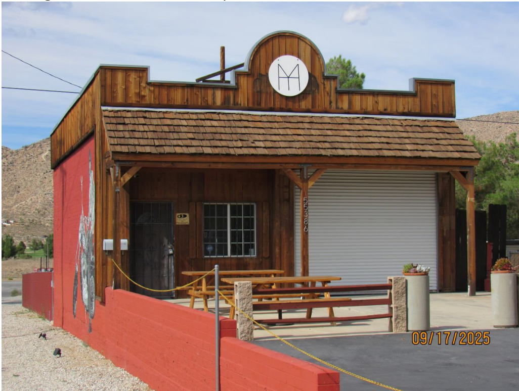
South Facing Wall
