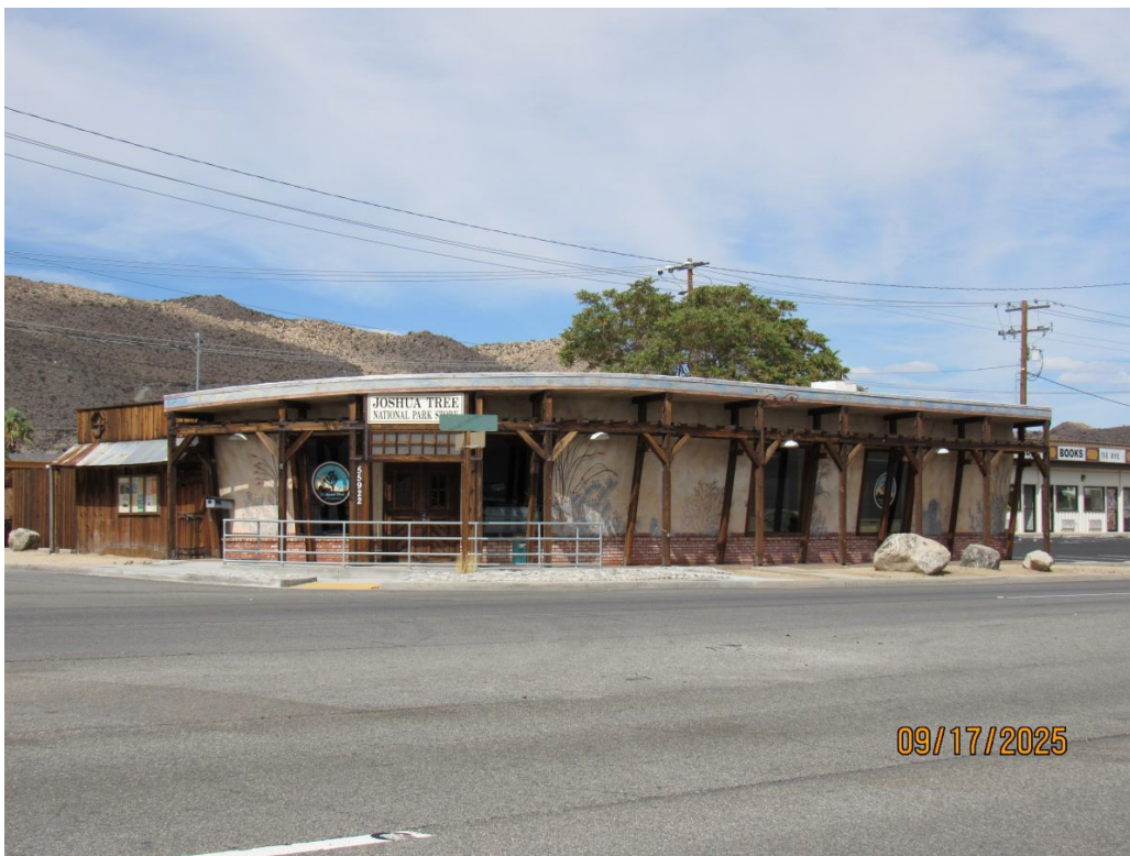
Southwest Corner Facing Wall
