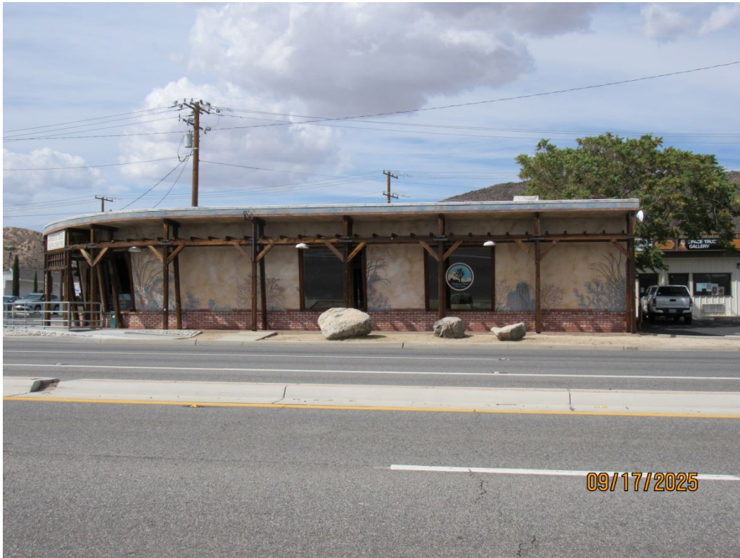
South Facing Wall
