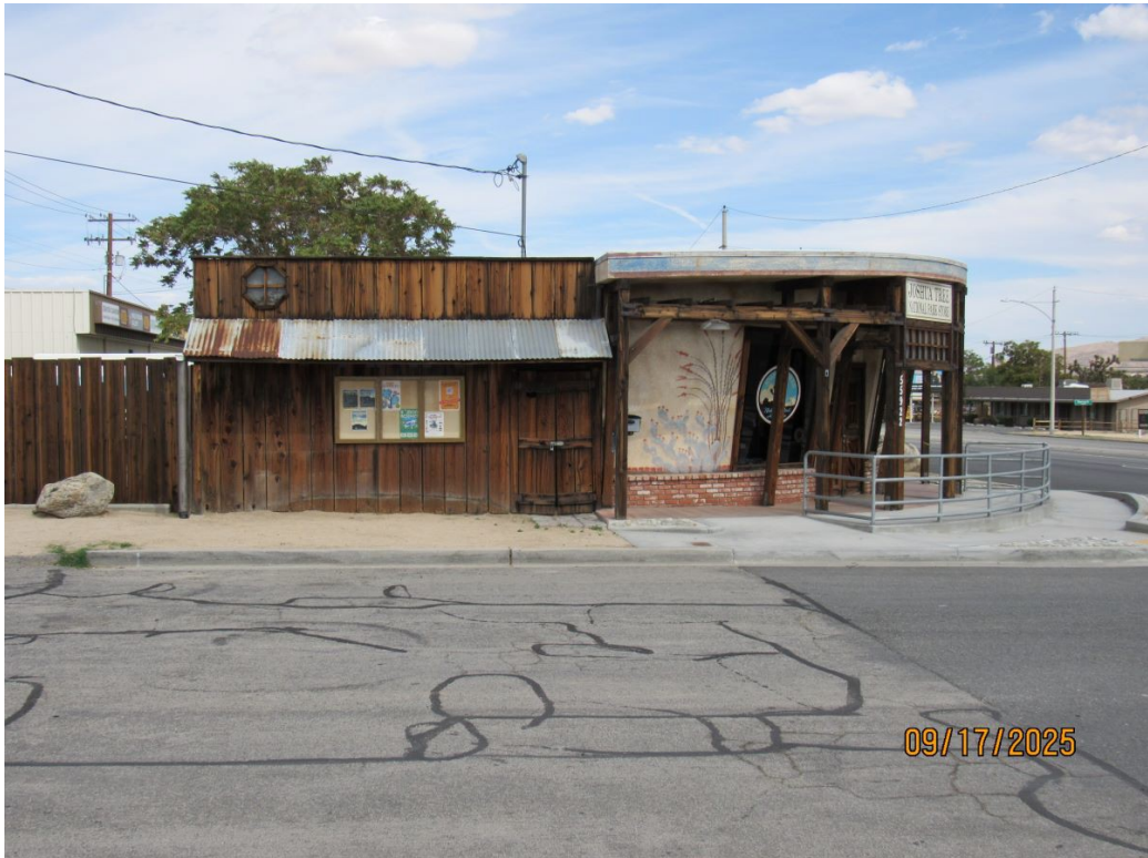
West Facing Wall
