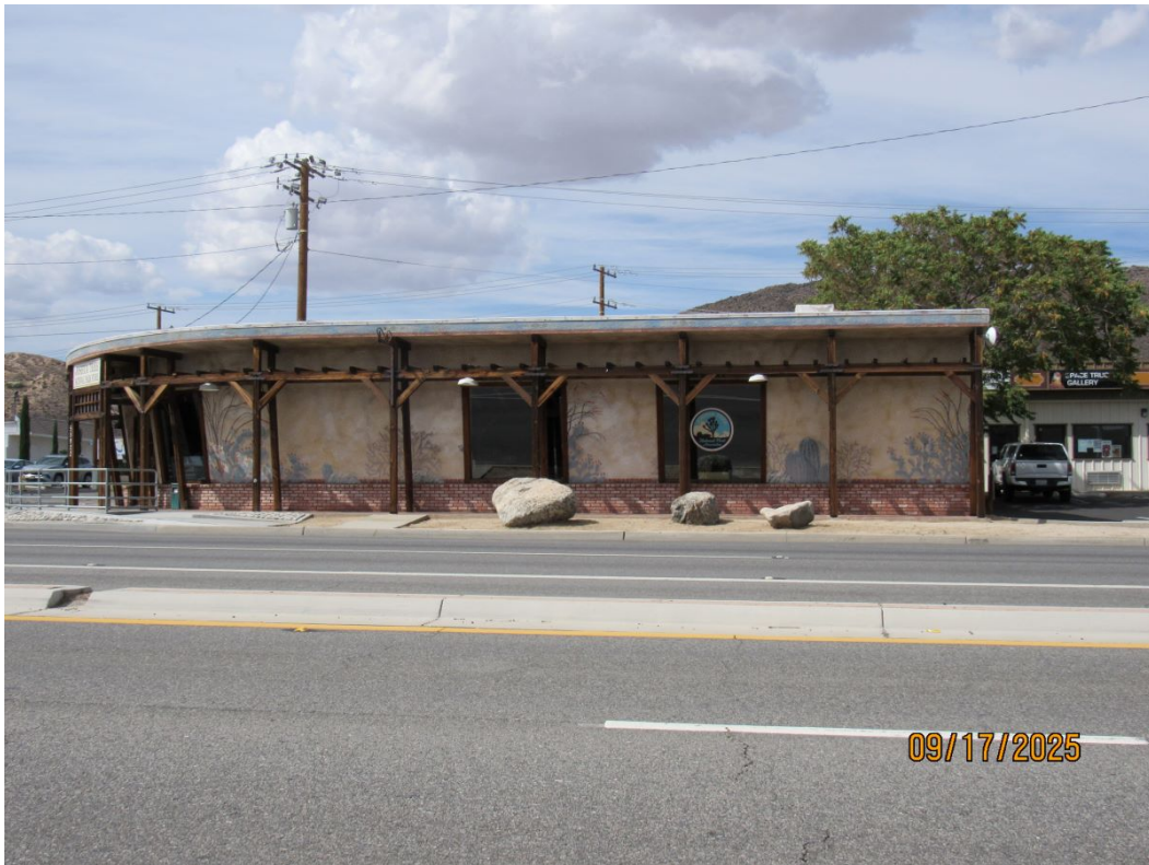
South Facing Wall
