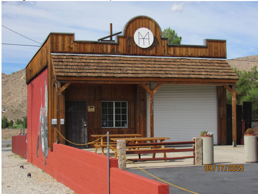
South Facing Wall
