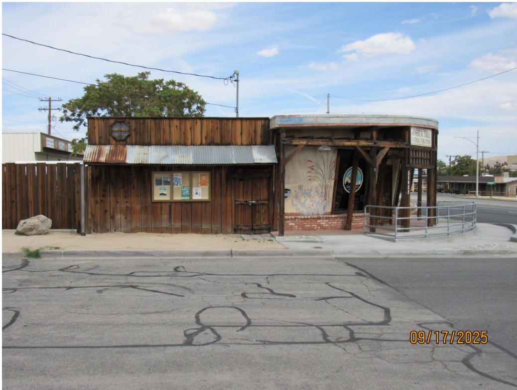
West Facing Wall
