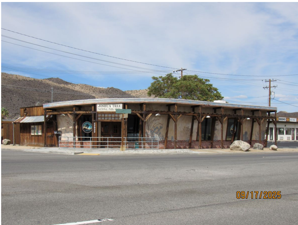
Southwest Corner Facing Wall
