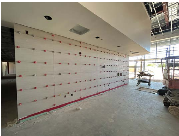
Wall Tile Install In Lobby
