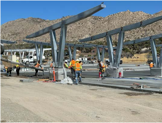
Concrete Paving North Parking Lot
