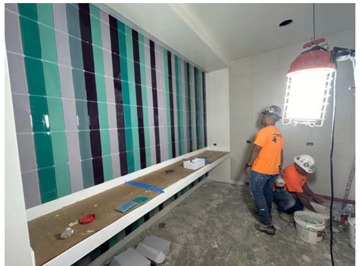
Wall Tile Install Men's Locker Room
